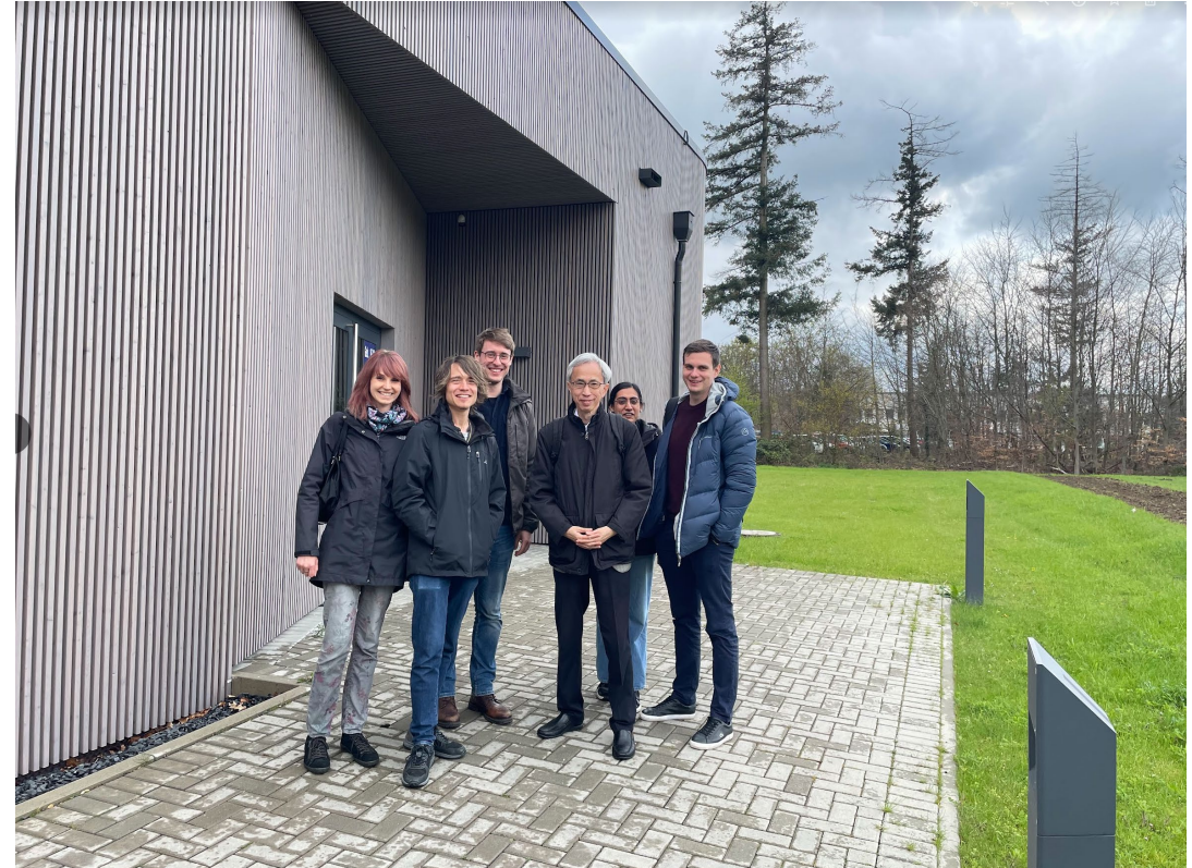
Building to house D-Wave Advantage
